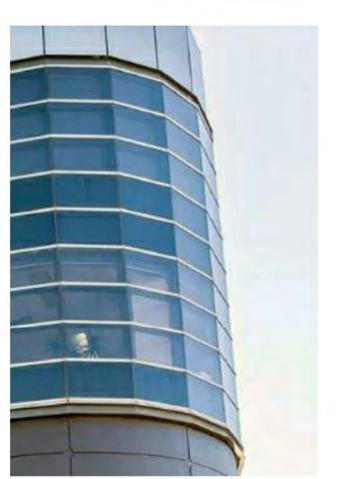
ED-02 CURTAIN WALL MATCH NEIGHBOURING BUILDING WITH A MIXTURE OF DARK TINTED GLASS PANELS (GL-01) AND OPAQUE PANELS (GL-02)
